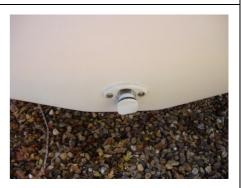
The seal is affected by an O Ring (Black ring in picture) on the plug that screws in, when the plug is removed inspect this O-ring without the O ring in place the bung will leak.
